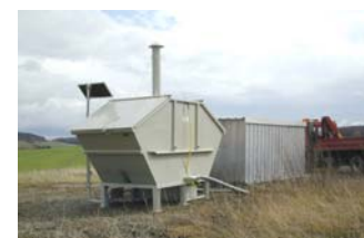
Passive venting system with bio-filter
