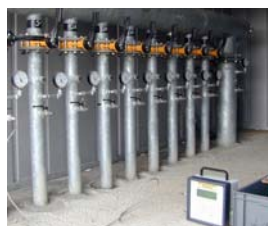
Gas drains merged at the central control bar
