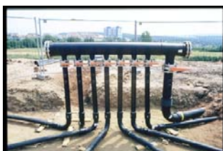
Gas drains merged at the central control bar
