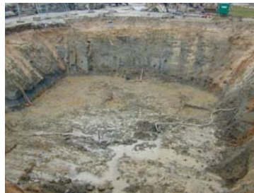
Cleaned-up excavation pit
