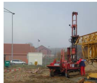
Drilling rig on a track vehicle
