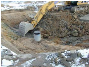
Excavating the contaminated soil
